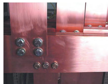
Double connection: 100 x 10 bars (3200 A) and 80 x 10 bars (2500 A) on 120 x 10 common bars
