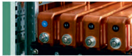
Example: the phases must at least be marked N, L1, L2, L3, at the ends and at the connection points.
