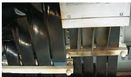
Clamping flexible bars
