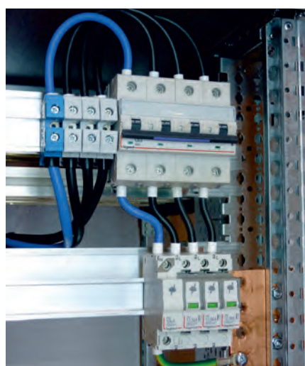
Another example of creating connections L1, L2 and L3.
